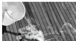
GENTLY WASH DECK WITH WOOD WASH
